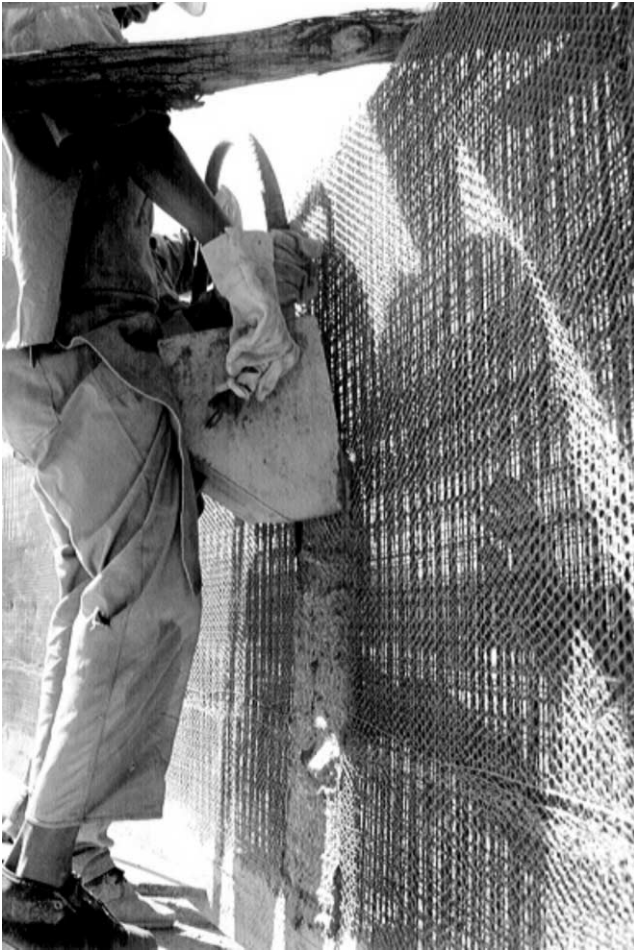
Fig. 1. Construction of ferrocement water tanks.
