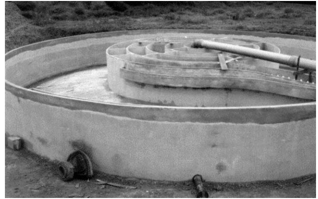
Fig. 2. Ferrocement water tank in Divinópolis, Brazil.
